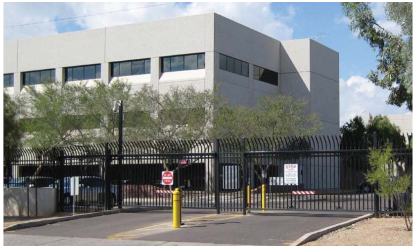
Ornamental iron security fencing and gates were installed at the DPS headquarters building to increase security.
